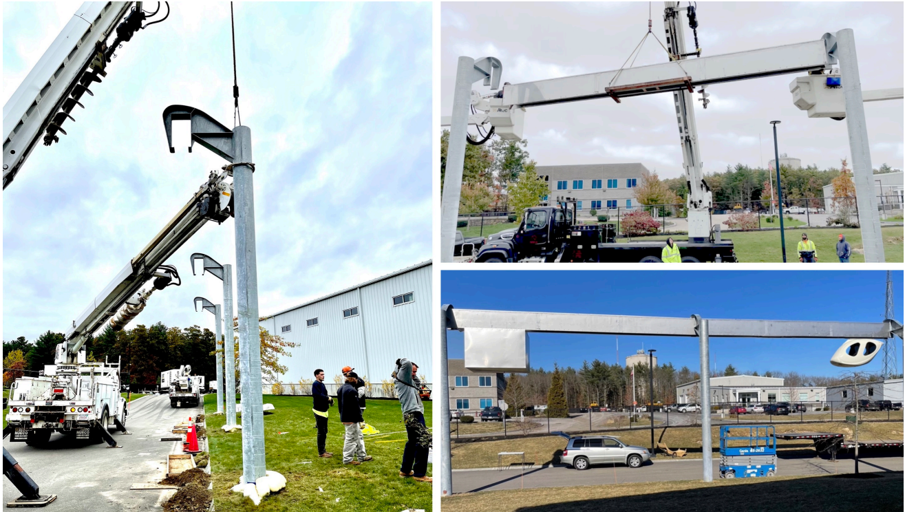
First Pilot Podway installation and testing
